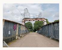
bridge. In 1967 the bridge was permanently fixed and the control cabin on top of the bridge was removed.
